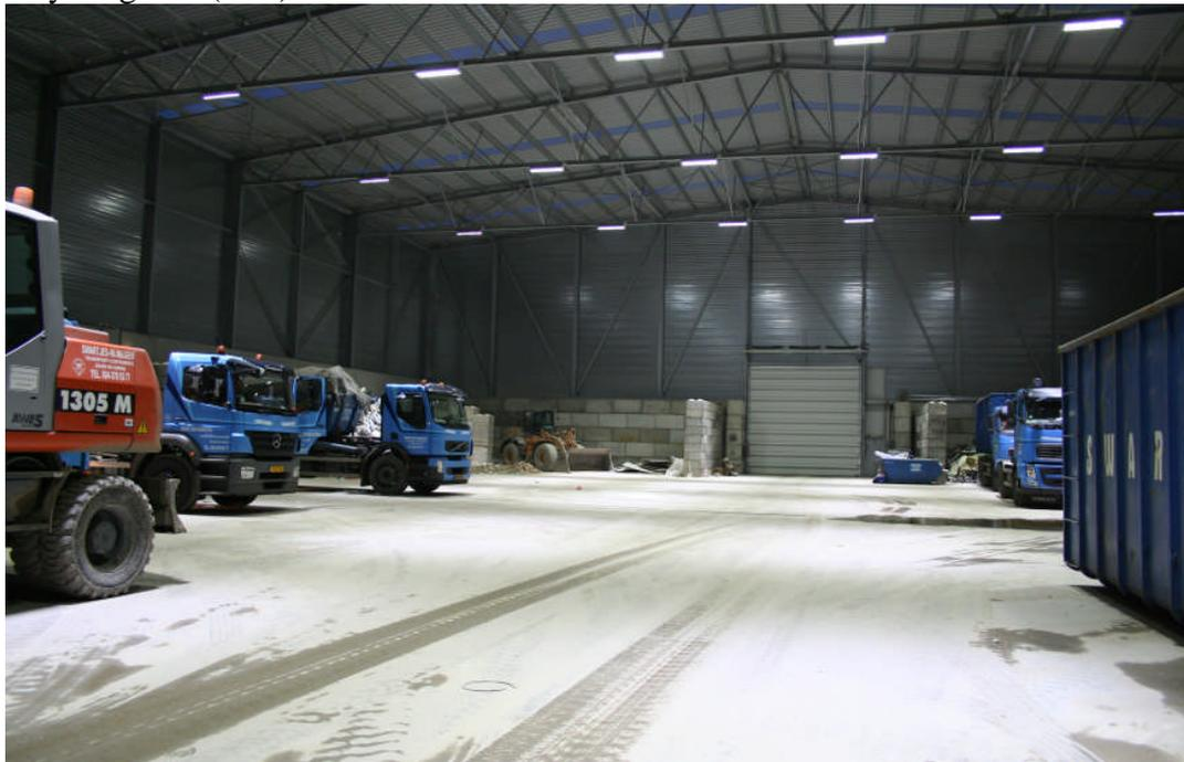
The lamps are at a height of 12 meters and the distance between the frames is 10 meters. The distance between the lamps, on the frames, is 5,5 meters and have been divided as 50,5 Watt – 4 times 101 Watt – 50,5 Watt . The amount of lux on the floor is 70-180 lux. To get 200 lux on the floor we need twice as much strips (101 and 202 Watt) but the principal is very satisfied (never had so much light) so pity they did not do.
